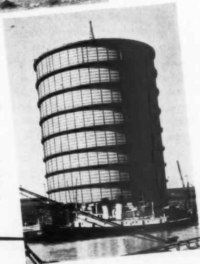
Largest all-welded, dry seal gas holder in the United States—10,000,000 cu. ft. capacity. Installed by Stacey Brothers Gas Construction Co., at Dearborn, Michigan.
